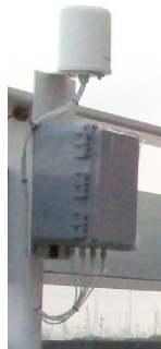
Outdoor MIMO Omnidirectional Antenna Installed With The 12" x 10" x 6" Polycarbonate Enclosure
