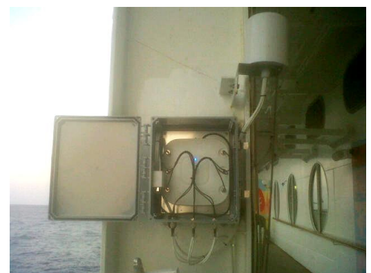
12" x 10" x 6" Polycarbonate Enclosure with Solid Door, Latch Locks, Cisco 3500 AP Series and Installed Outdoor MIMO Omni Antenna
